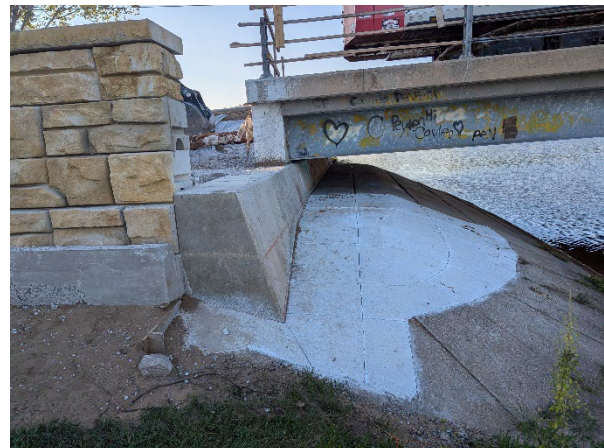
Completed abutment ready for steel beams
