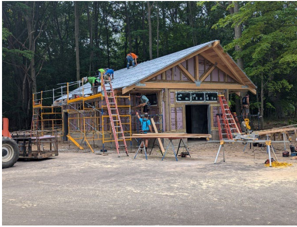
Day Use Restroom in progress
