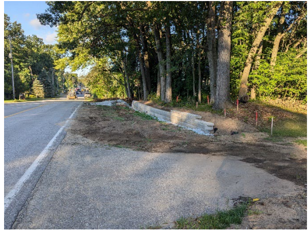
Trail construction east of bridge
