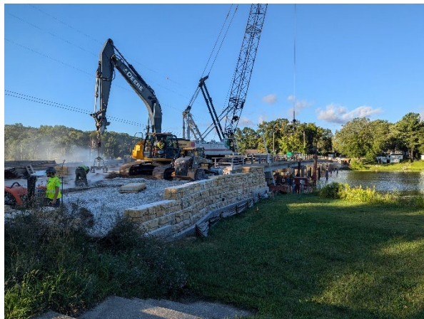
Bridge construction in progress
