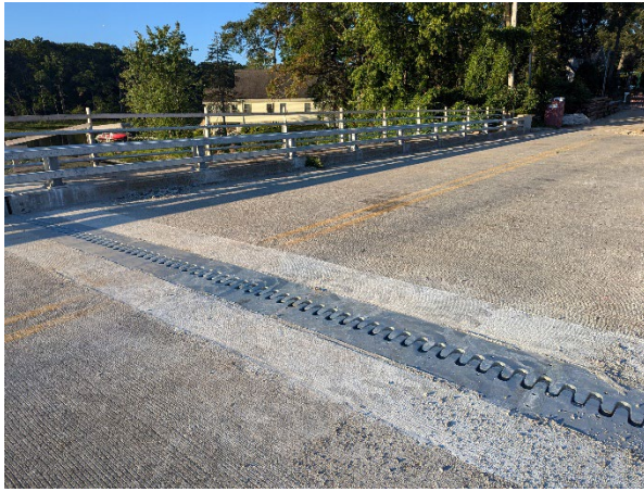
Bridge joints and south railings nearing completion
