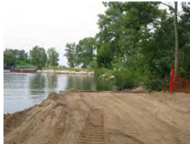
Boardwalk approach looking west
