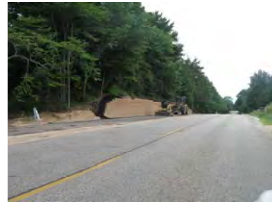
New Retaining Wall
